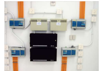
Vesda Early Warning Smoke Detection System
